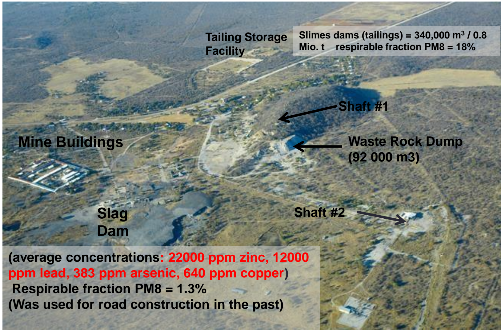
Aerial View of Berg Aukas Looking Northeast
